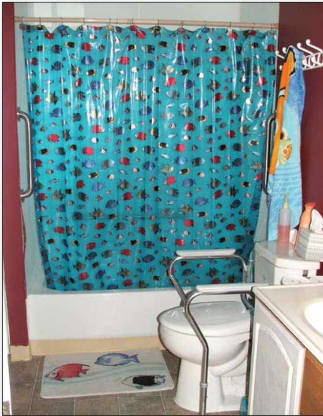
Bathrooms in the Senecal home were retrofitted with grab bars and ADA raised height toilets
